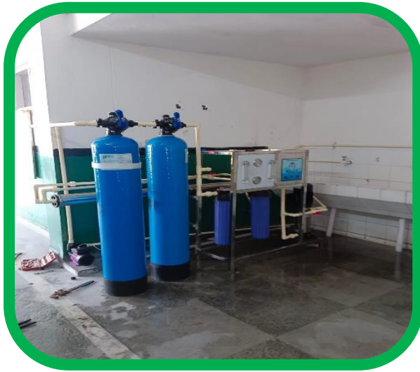
03 XRO plant Installed
