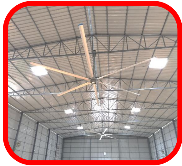
02 X HVLS Fans fitted in MPH
