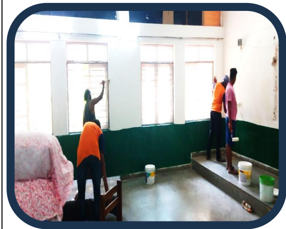
All rooms are Distempered
